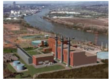
Image of the Bethlehem Energy Center - PSEG Facility
